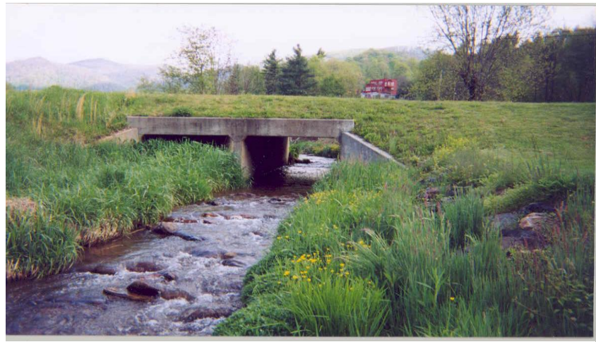
Figure 3. Culvert with Floodplain Bench
